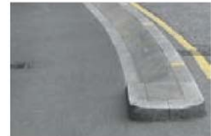
Use of shallow angled battered kerb to increase effective width, London
