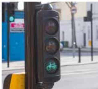
**Figure 31. Junctions** – Low level signals – the Statutory Instrument Traffic Signs Regulations and General Directions now permits measures that can support older cycling (Photo: Sustrans UK)
